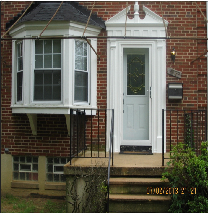
TYPICAL End of Group Covenant Compliant Home Front Entrance Door Trim Two Original Design Fluted Pilasters and One Plinth Block on each side, Acorn Pediment, Standard Crosshead with 6 Fluted Teeth.
